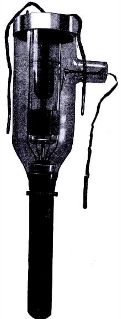
Here is the No. 507, water cooled, 10,000 watt transmitting tube.
